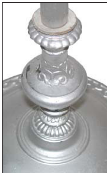
Close up view of the ornamental, cast-iron base.
