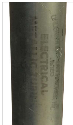
Detail of a tube, stamped with “UNDERWRITERS LABORATORIES, INC. / LISTED / ELECTRICAL METALLIC TUBING.”
