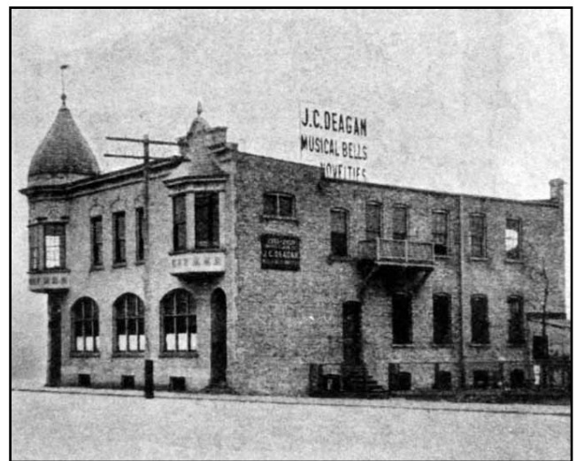
Figure 3. Deagan’s factory occupied this structure, complete with his name on the roof, between 1904 and 1912. It indicated the size to which his manufacturing business had grown in two decades. Author’s collection
