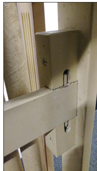
Detail of the wooden rail joint on the inside of the end board showing the pegged tongue-and-groove construction.
