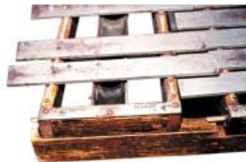
Detail of the frame showing Deagan’s name, company location, patent dates, and the bar mounting system using felt and cord.
