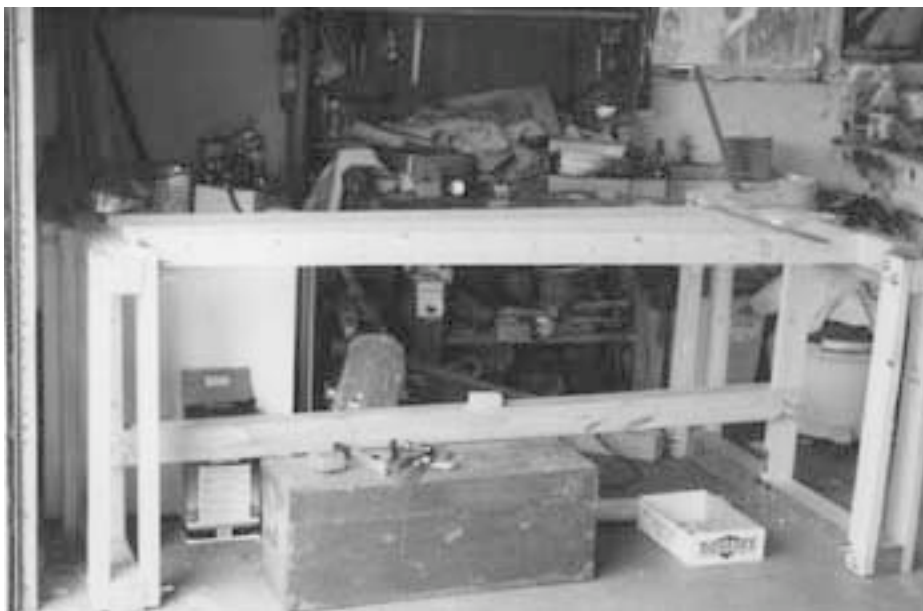
PHOTO 3—The frame, freshly put together.
