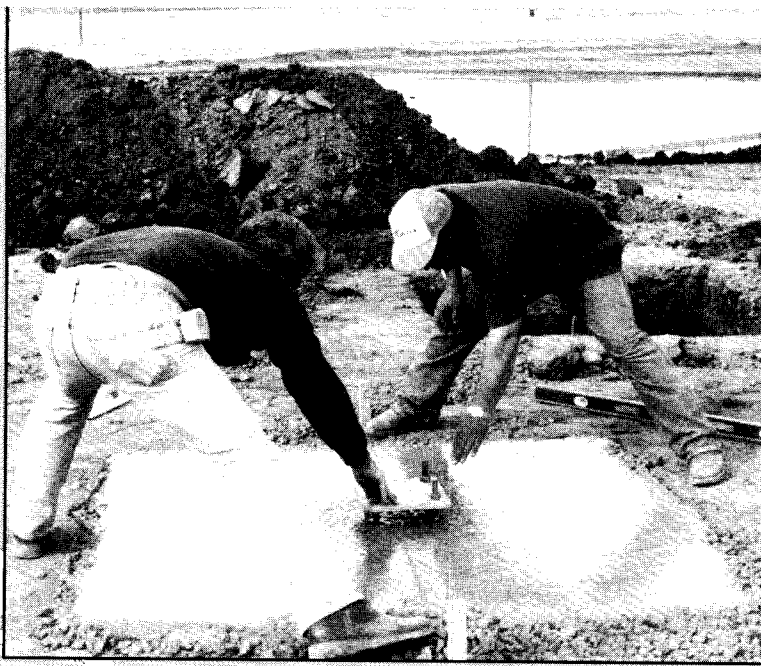
Then workers performed backfill and soil compaction of the spread footings.
